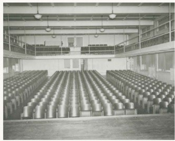
Farmville High School Auditorium, Plaintiff's Exhibit No. 14
